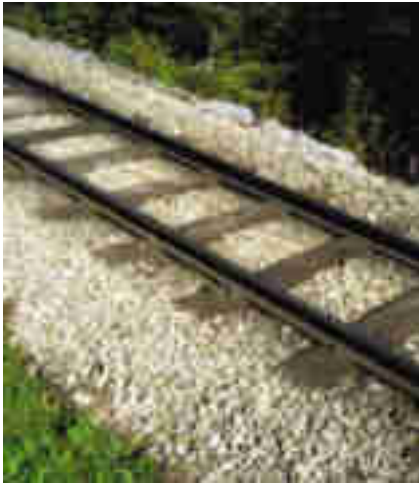
Real railroads, like Switzerland's BLM line, float their track in a bed of ballast.
